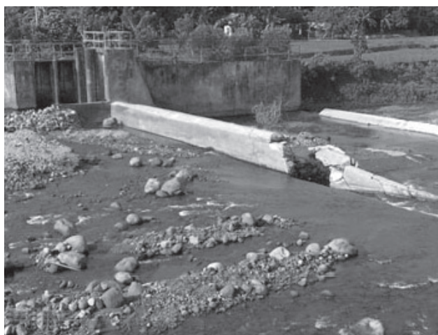
Picture 1: Bukas Mata CIS Dam, broken in a typhoon and awaiting funds for repair.
